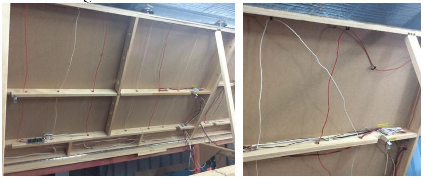
• And then run smaller feeder wires from the track to the Bus wires.
